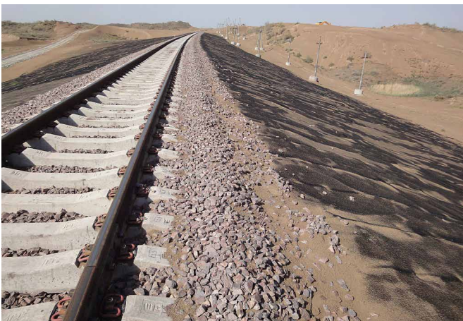
(fig. 5) EnkaMat 7018 application in desert area to prevent wind erosion with high UV-exposure (project Kazakhstan)
