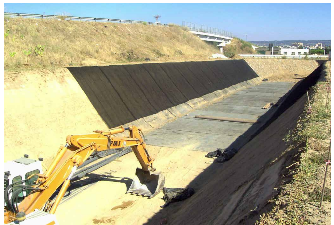
(fig. 6) EnkaMat 7220 application storm water channel with high UV-exposure in dry season (project Taranto South Italy)
