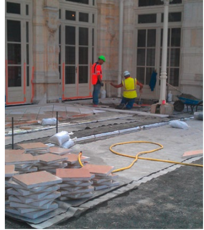
EnkaDrain® V-shaped under (sealed) pavings
