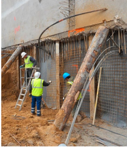
EnkaDrain® B10 for drainage behind shotcrete
