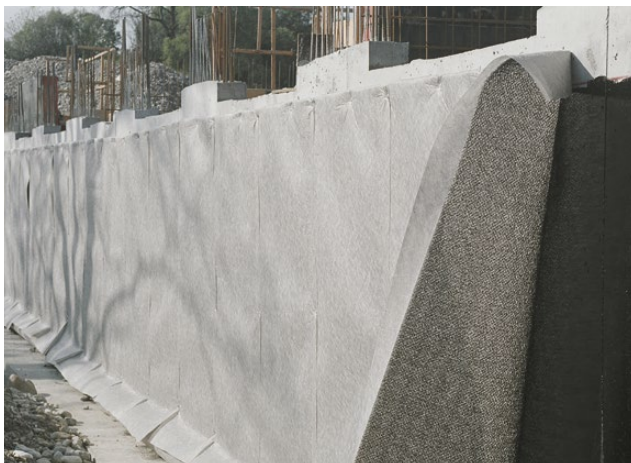
Vertical drainage on basement walls
