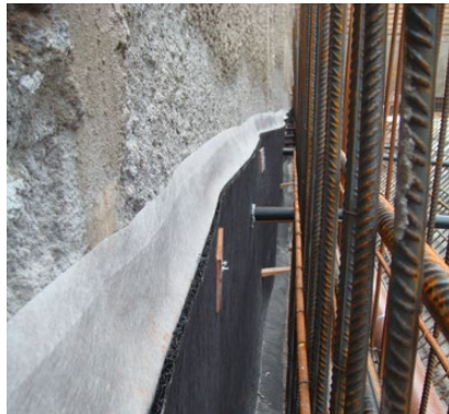
EnkaDrain® CKL as lost shuttering on diaphragm walls
