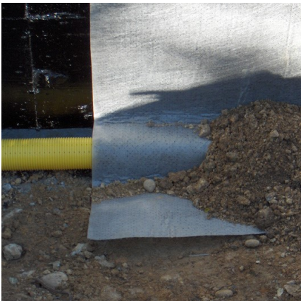
EnkaDrain covers the pipe to protect it from clogging.
