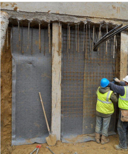
Bottom overlap for shotcrete applications.
