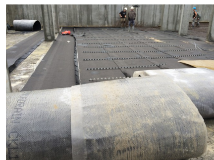
For EnkaDrain CKL, the black fleece has to be faced upwards (i.e. faced to concrete slab).
