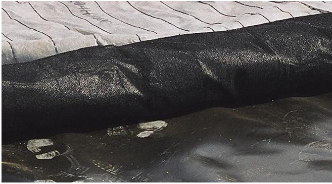
The drainage core of EnkaDrain Wide with one fleece only “-1s” has to be faced to geomembrane, i.e. downwards for rainfall or leachate drainage and upwards for gas pressure relief.
