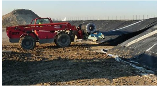
On slopes, rolls must be unrolled with care from the top to the bottom of the slope.
