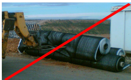
Use an appropriate device for unloading and handling of the rolls
