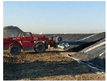
Fig. 10 – On slopes, rolls must be carefully unrolled from the top to the bottom of the slope.
