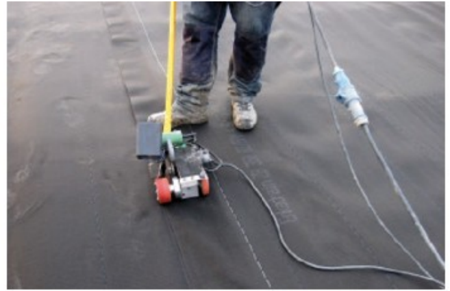
Fig. 12 – Spot-welding with a hot-air device.
