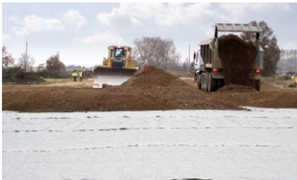
Fig. 1 – Drainage/Filtration under road embankment
