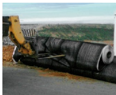
Fig. 4 – Handle with care. Use fork-lift device with a central pole to prevent damage
