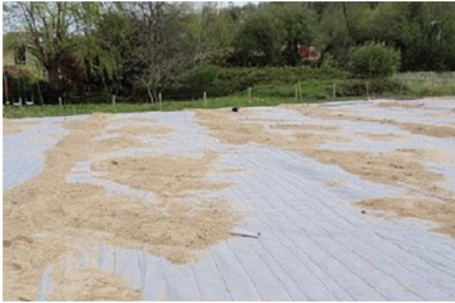
Fig. 11 – Prevent rolls and overlaps being displaced and opened by wind or traffic. Cover or weigh down with appropriate materials (heaps of soil, ballast bags).
