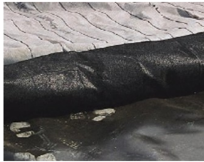
Fig. 9 – EnkaDrain Wide “-1s” laid on rigid material with its core downwards for rainfall drainage.
