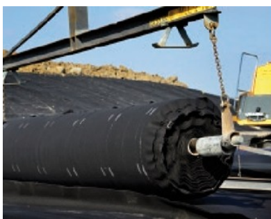
Fig. 3 – Appropriate devices must be used for unloading and handling the rolls
