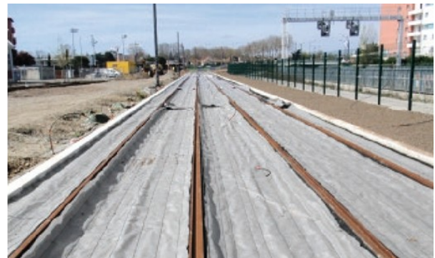
Fig. 2 – Drainage/filtration on tramway platform
