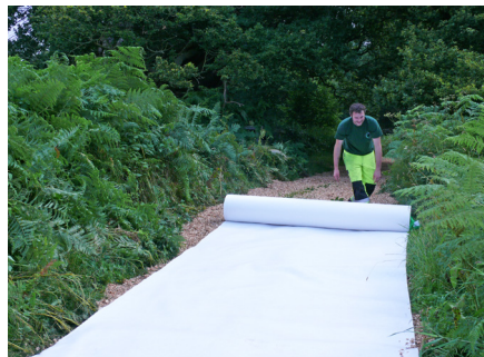
Lay Geotextile
