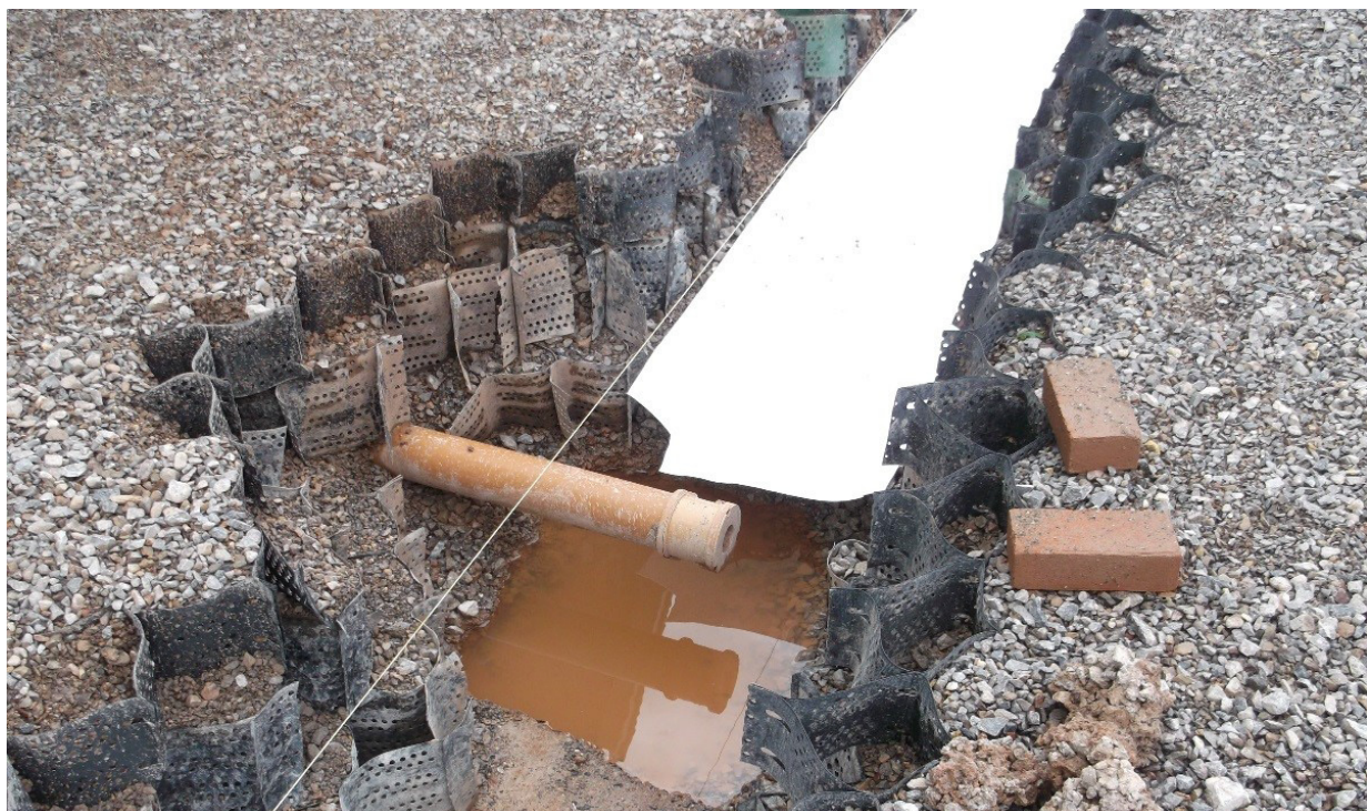
Image 2. Cellweb alongside drainage pipe
