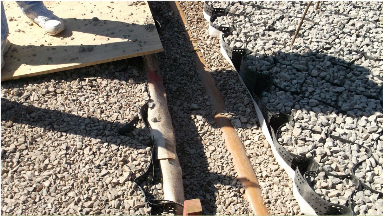
Image 1. Cellweb alongside drainage pipe
