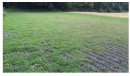
Turfmesh 4 suited the grass car park due to the soil conditions and numbers of vehicles using the site. With the help of volunteers and assistance from Geosynthetics Ltd, the Turfmesh was installed at the start of July 2016.
