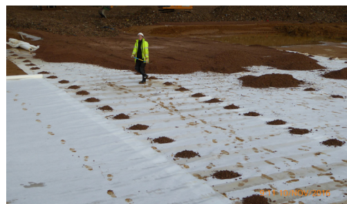
Ekotex 14 being installed
