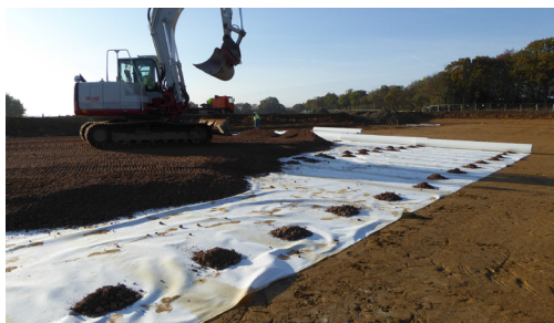
Ekotex 14 being covered by subsoil
