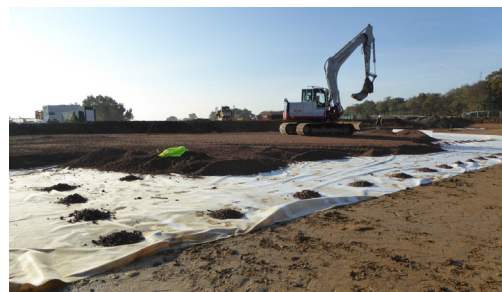
Ekotex 14 being covered by subsoil
