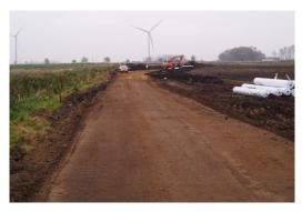
The 80m diameter wind turbine blades at Stags Holt are mounted on 59m high towers. Each turbine can be accessed by approximately 8km of internal access tracks that is approximately 5 metres wide, with areas of hardstanding adjacent to each turbine for use by cranes during construction.
