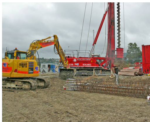
Platform supporting SF20 Rig and Tracked Plant
