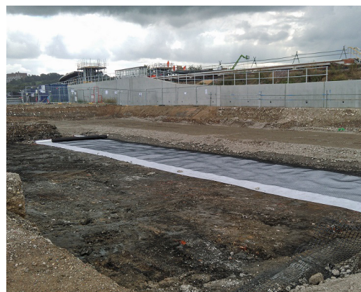
Base layer of Tenax HM4 and Ekotex 07 Separation layer
