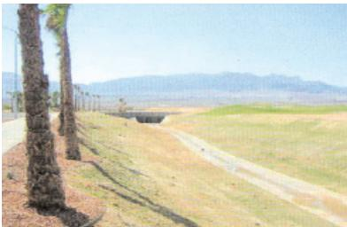
Tan coloured Pyramat® lines a channel running through a residential development in the Southwestern U.S. Reinforced concrete was originally specified for the project, but use of the HPTRM resulted in savings of approximately \$1.2 million (U.S.)
