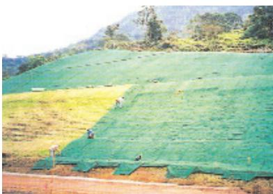
Landlok® TRM's are ideal for providing protection and vegetation reinforcement on steep slopes.
