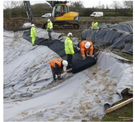
rolled in very compact packages – one for each pond and apron; labeled accordingly. ii. The Aquablock® was pre-fabricated into a single piece for each pond – no onsite jointing was required; it could be simply unrolled and unfolded across the ponds. iii. We delivered all three liners to site just 5 working days from the initial order. Over 1,600m² of product made to order within a
