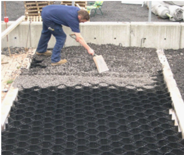
Figure 2 - Cellweb TRP® in construction.
