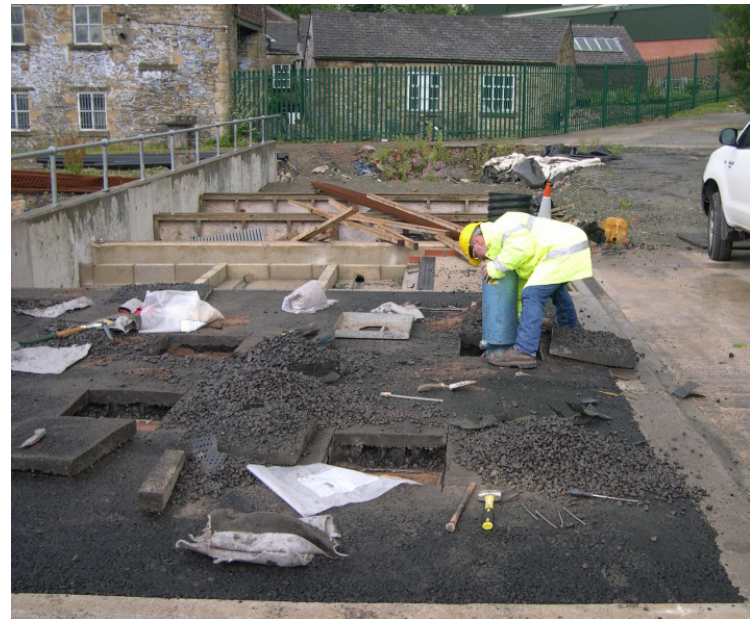
Figure 3 - In situ density tests post-trafficking.
