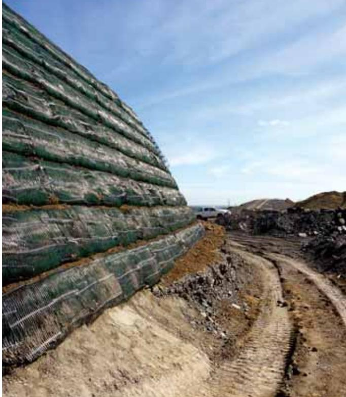
FIGURE 7 Construction of the gabion wall on top of the RSS. Photo: Geosynthetics Ltd.
