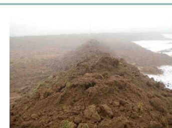
7 Putting the required 300mm of cover over Bentotex using as dug material
