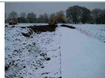
6 Laying the Bentotex in the snow
