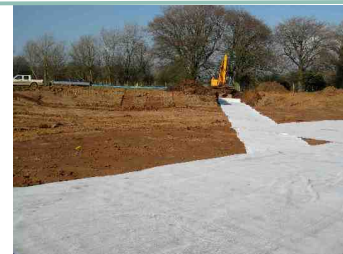
3 Maneuvering and laying Bentotex with a 'spreader bar'
