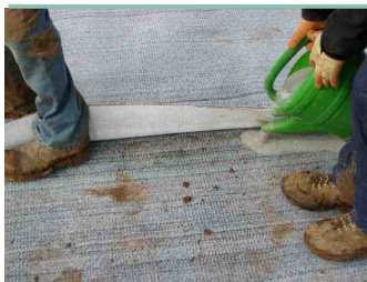
5 Laying the Bentotex granules to seal the laps.
