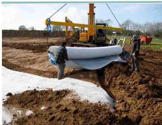
3 Maneuvering and laying Bentotex with a 'spreader bar'
