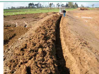
2 Digging Anchor Trench
