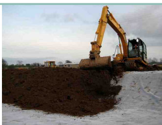
7 Putting the required 300mm of cover over Bentotex using as dug material
